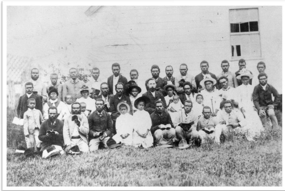
Plate 11.17: Rev. McIntyre and the congregation of the Presbyterian Mission at Walkerston. There are seven children in the photograph.
