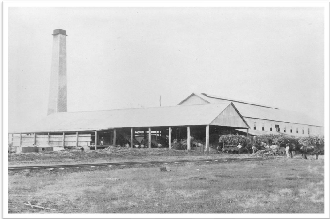
Plate 10.15: North Eton central mill, 'The Defiance', first crushed in 1888. This photograph is from 1895.
