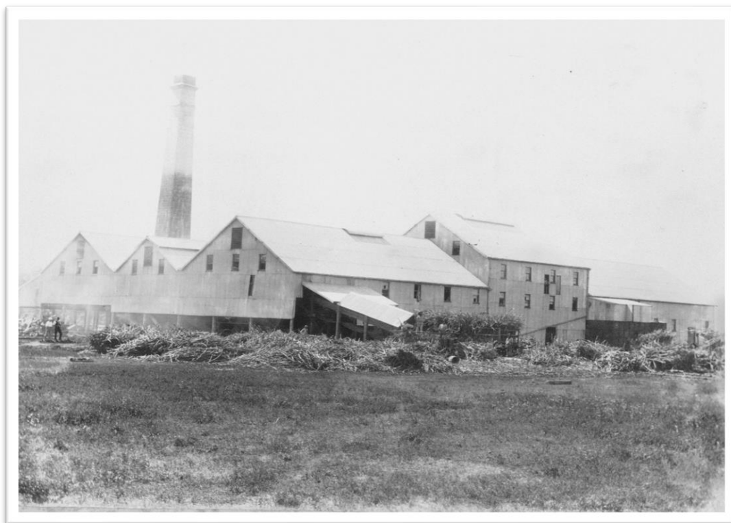
Plate 10.12: Racecourse central mill which first crushed in 1889.
