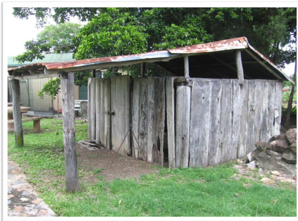
Plate 6.7: The Hamilton structure was moved and is now part of Mirani Museum, labelled as a ‘dairy’. Some of the defence holes are visible in this photograph.
