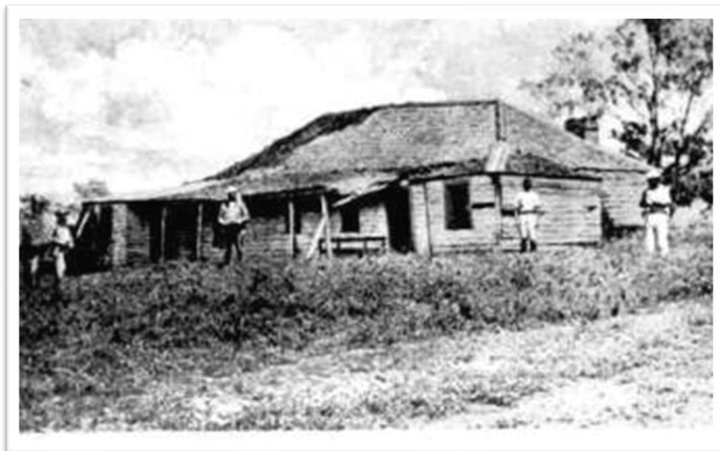
Plate 4.3: The first Turanville station homestead at Scone, demolished in the 1860s to make way for the new house. Thomas Cook, F.H. Murray and a station hand are standing in front of the house. The increase in wealth is obvious when comparing this house with the new homestead below (Plate 4.4).
