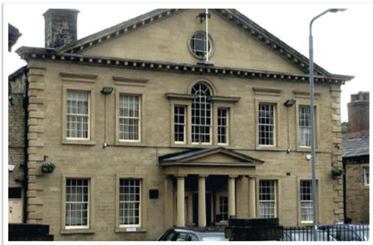
Plate 5.29: Stoney Royd or Somerset House in Halifax, built between 1762 and 1765 for John Royds, a merchant in the textile trade. It is near the town centre. The front (in the photograph) was once the back. The original front had gardens which swept down to the Hebble Brook. Wings on both sides of the main house were once used as stables and a warehouse. It was sold in 1807 to William and John Rawson for use as a bank, which it remained until 1898. It was the Huddersfield Building Society, then the Halifax & Huddersfield Union Bank, but often called Rawson's Bank. It is now the Albany Club. The warehouse and stables wings of the house were sold separately.
