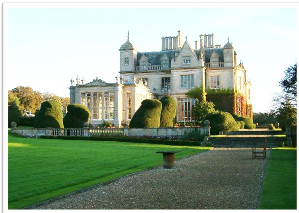
Plate 5.18: Stoke Rochford Hall in Lincolnshire, home of Christopher Turnor, an investor in Mt Spencer station. He was married to a sister of Henry and Harold Finch-Hatton. His son Graham owned Bolingbroke station, near Mt Spencer. Source: Courtesy of Patrick Mackie, CC BY-SA 2.0, https://common .
