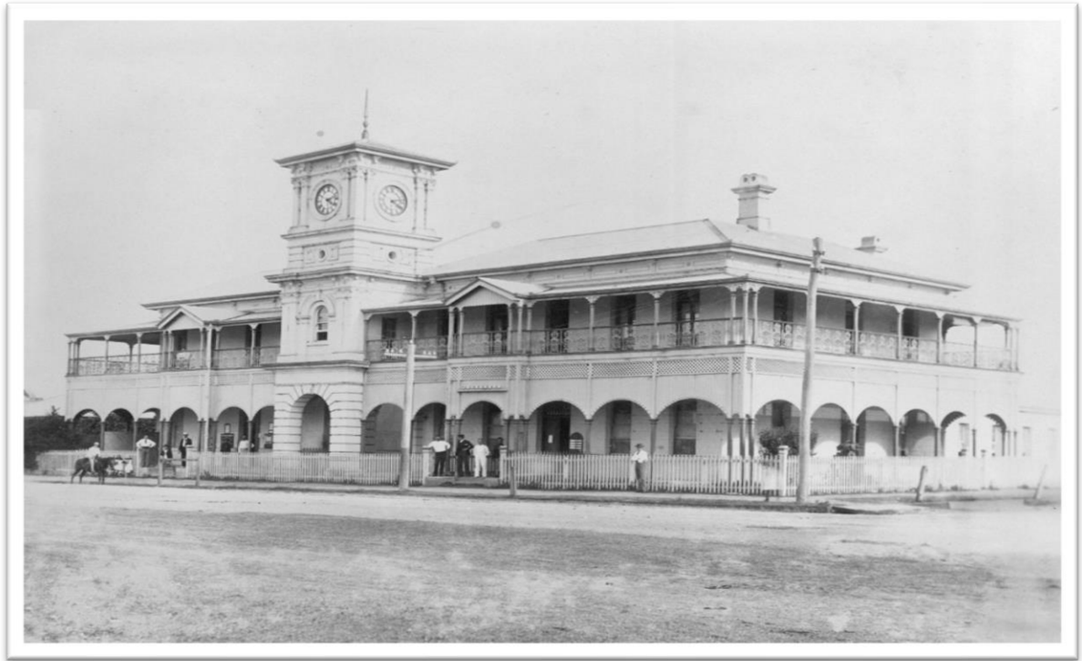
Plate 14.22: The completed Post and Telegraph Office in North Street. The Postmaster's residence is in the upper story. The clock tower, used to regulate time at Mackay, replaced the Council clock. Source: State Library of Queensland.
