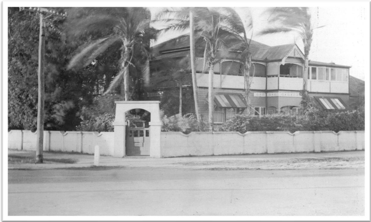
Plate 14.45: Dr C.E. Williams' residence on the corner of Albert (Gordon) and Brisbane streets. Source: State Library of Queensland.
