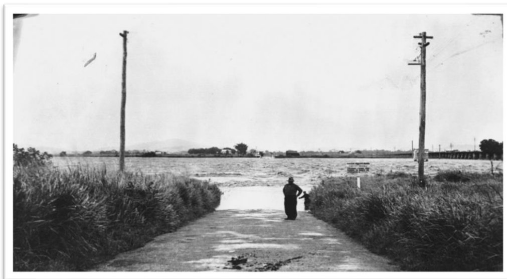
Plate 14.71: In this undated photograph the Pioneer (Hospital) Bridge over the Pioneer River has disappeared under floodwaters.
