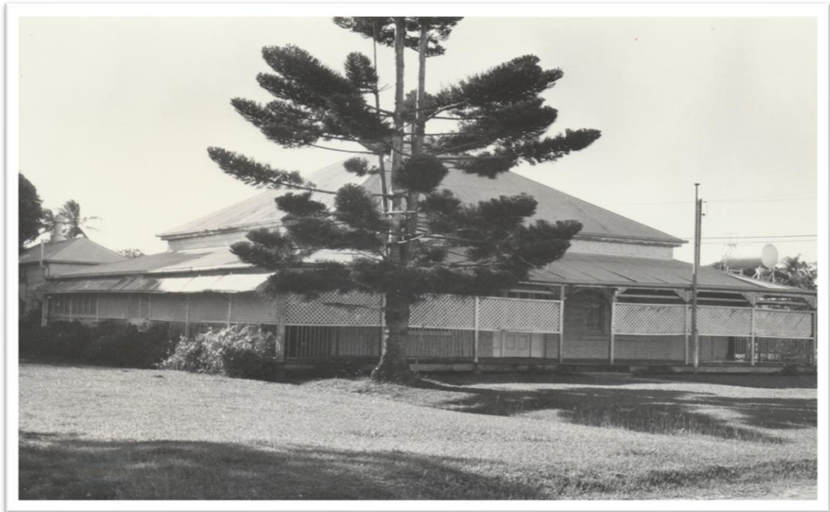
Plate 14.48: The Hamilton family home in James Street in 1979. The lattice screens around the verandahs are typical of the grand late nineteenth century houses. Source: Clive Moore Collection.
