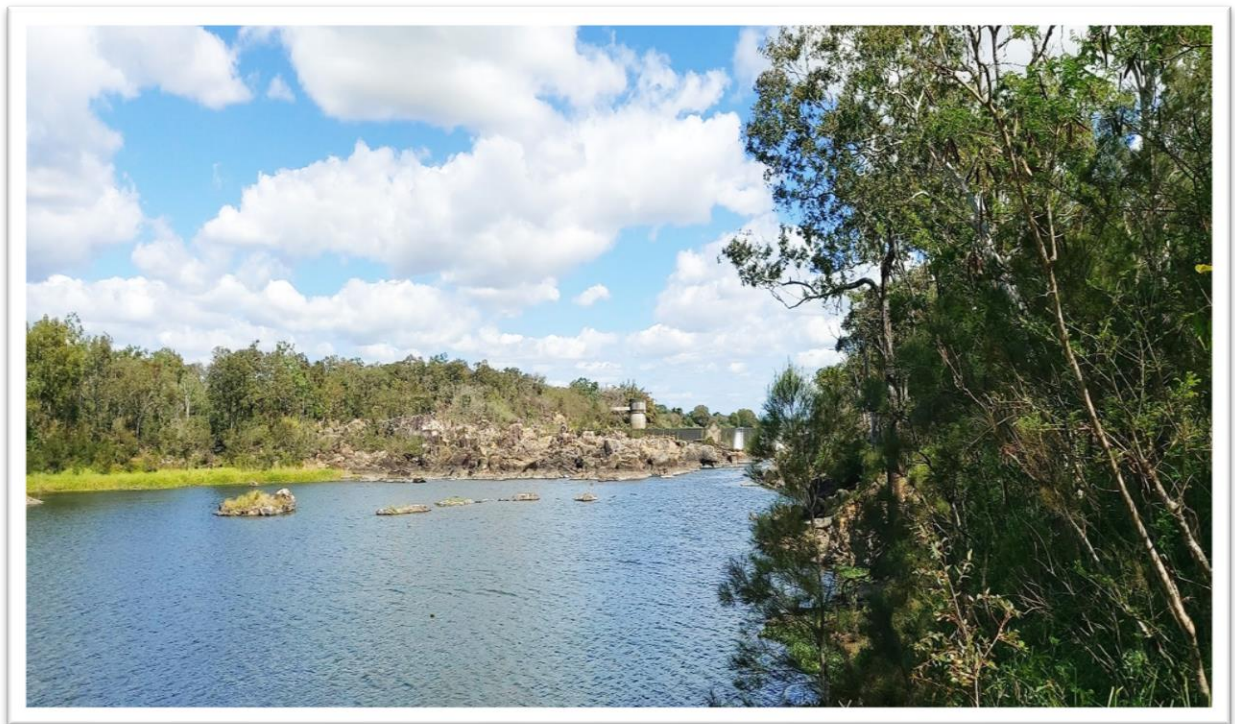
Plate Intro.17: The Pioneer River has several weirs and dams: Marian Weir was built in 1952, followed soon after by Mirani Weir. Dumbleton Weir (pictured here) was built in 1982, 15 kilometres upstream of the river mouth, at the point where the saltwater stops, and the fresh water begins. Dumbleton Weir provides water for Mackay. It has been upgraded twice. In 1977, water from the Pioneer River was diverted into Kinchant Dam between Mirani and Eton on the upper reaches of Sandy Creek. Teemburra Dam was constructed in 1997, 50 kilometres west of Mackay at Pinnacle.
