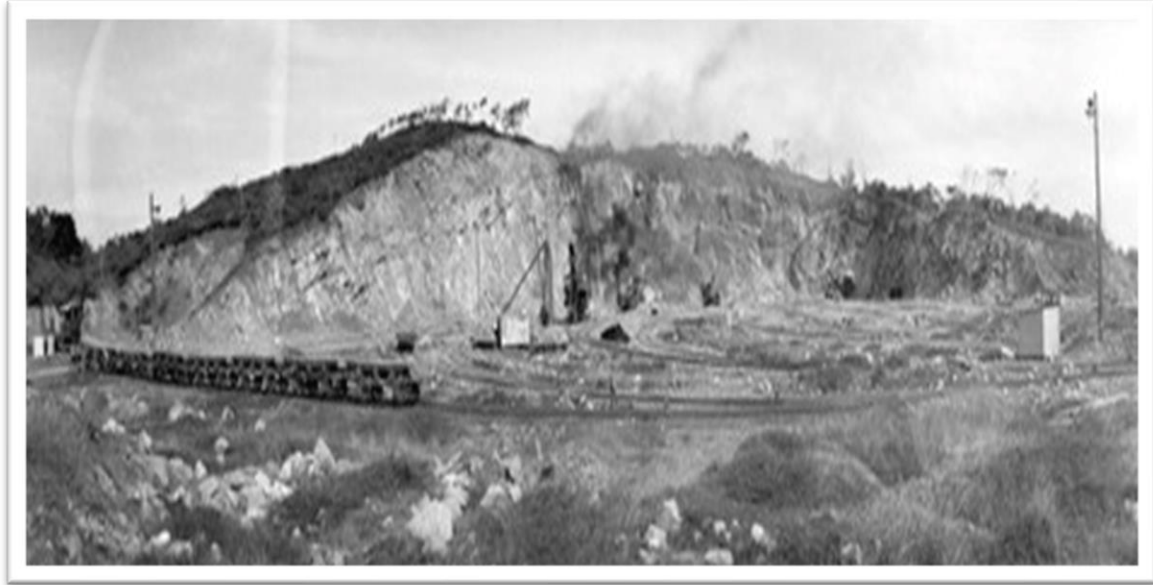
Plate 13.14: The mining of diorite from Mt Bassett quarry, used to create the outer harbour. Source: State Library of Queensland.
