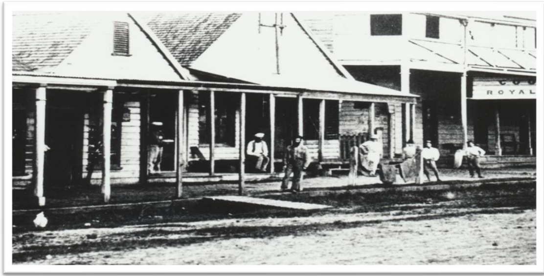
Plate 13.30: Enlarged from Plate 13.29. This is the adjoining building to Jane Cook's Royal Hotel in Sydney Street, 1870s.
