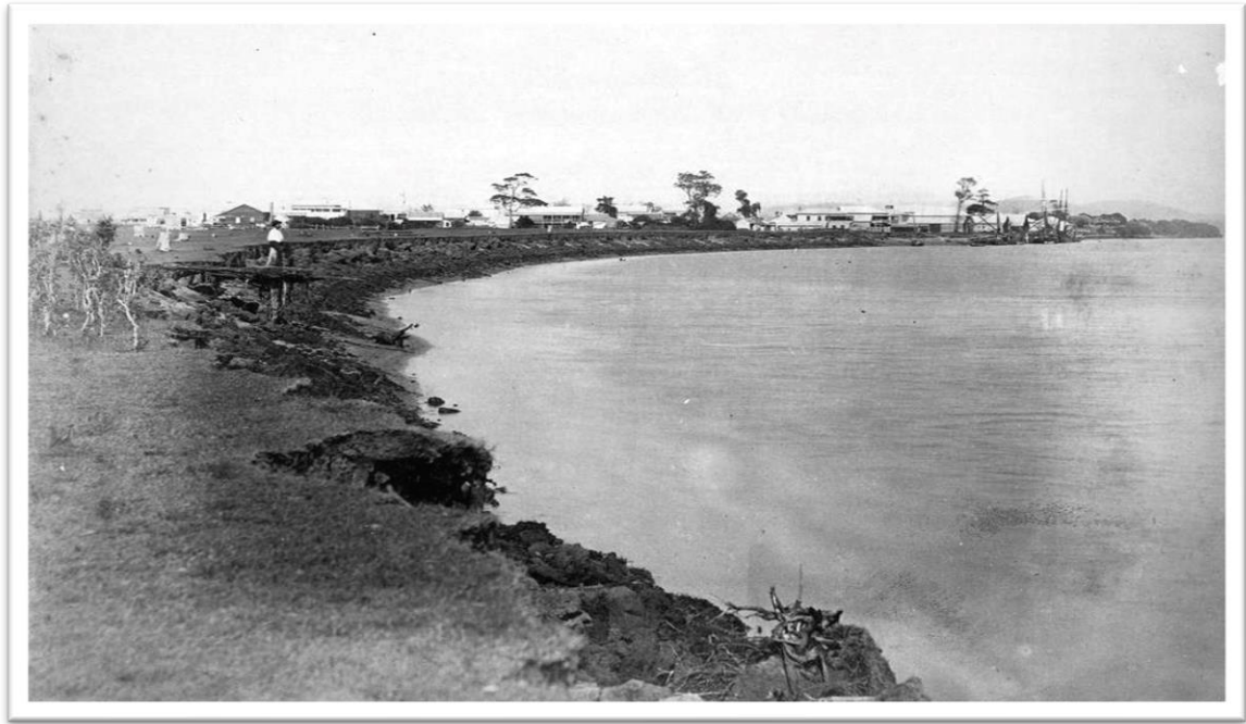
Plate 13.8: The banks of the Pioneer River were constantly eroding and difficult to use as a major port. This 1870s photograph, taken from the coastal end of the town, shows the early wharves. The river is tidal and was always too shallow to berth large vessels.
